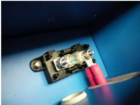
48V battery – double cable Double battery cable to fuse holder 200A fuse
